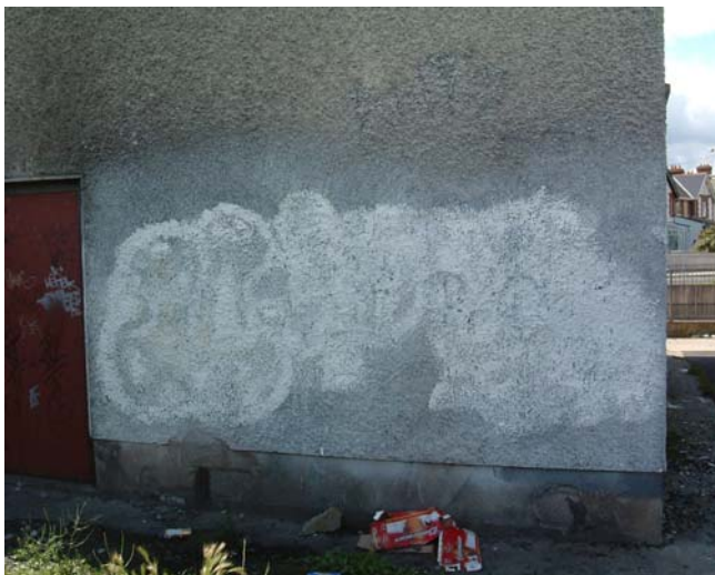
Spot covering - not recommended
