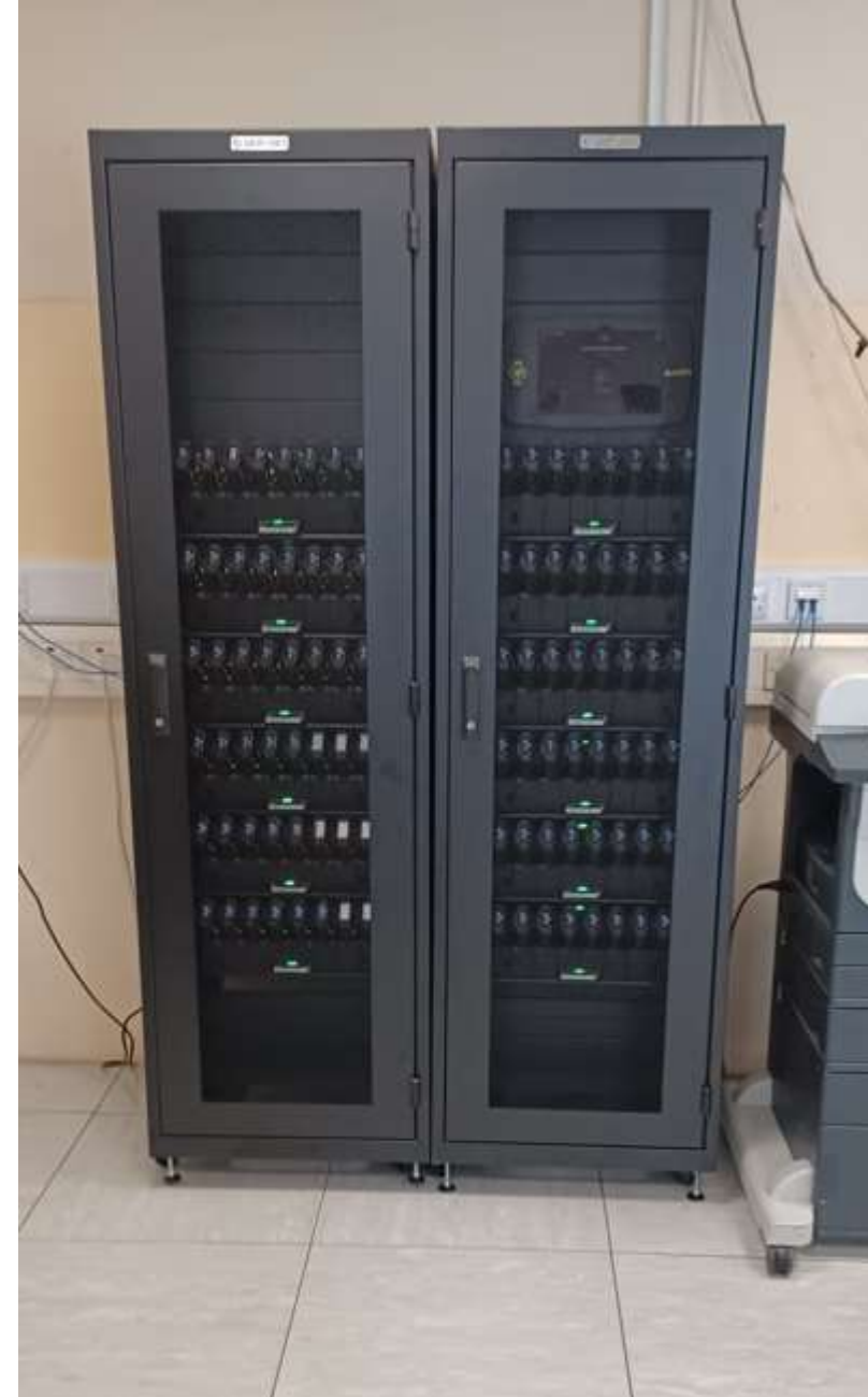
Store Street – 100 Cameras
