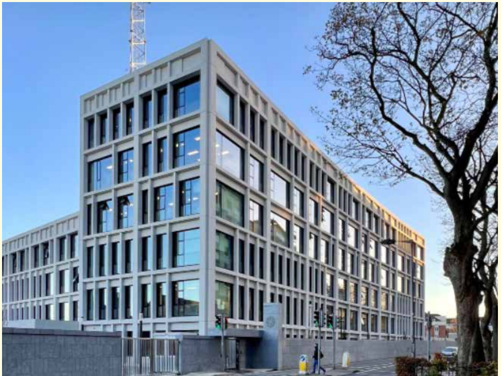
Walter Scott House, Military Road, Dublin 8.
