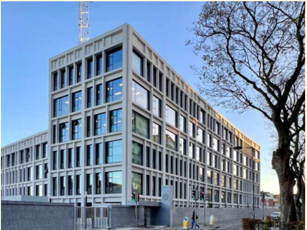
Walter Scott House, Military Road, Dublin 8.
